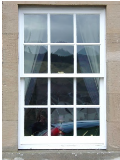
Figure 15: 6 on 6 Sash & Case Window
