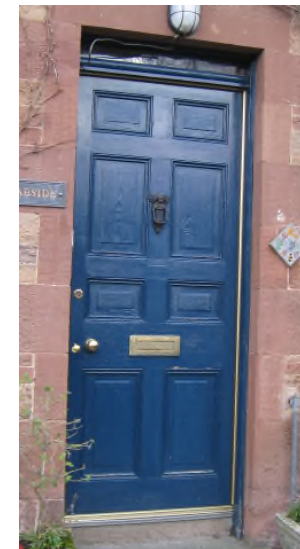
Figure 24: Example of a Panelled Main Entrance Door
