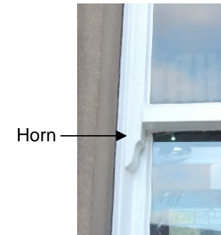
Figure 18: Traditional Window Detail - Horn Detail
