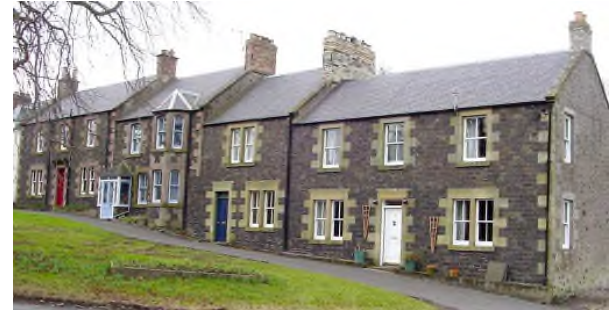
Figure 2: Historic Street Frontage - Yetholm
