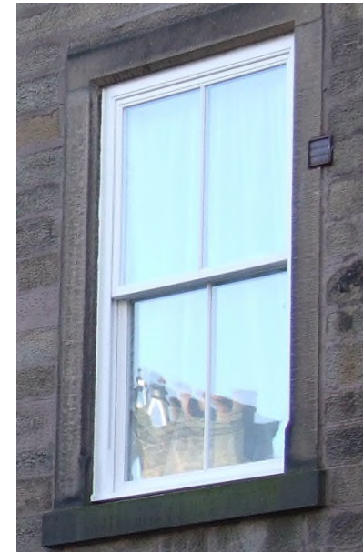
Figure 22: Acceptable Replacement Window
